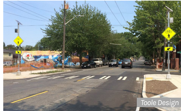
RRFB at a neighborhood bikeway crossing
