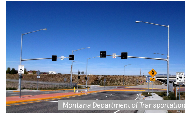
A pedestrian hybrid beacon in Belgrade, MT
