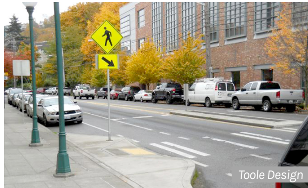
Mid-block curb extension
