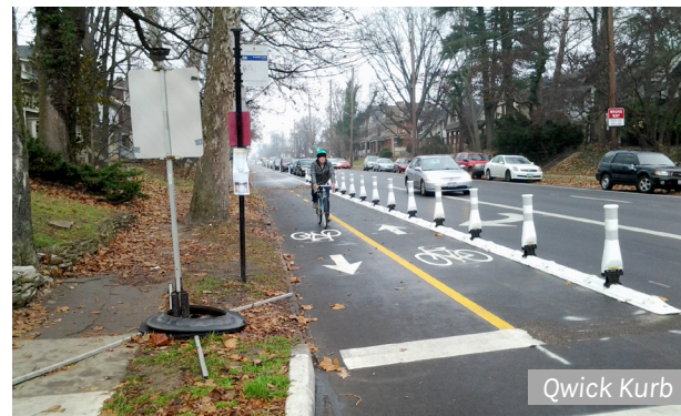
A two-way protected bike lane with temporary pin-down curb
