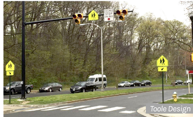
Pedestrian hybrid beacon on a divided roadway
