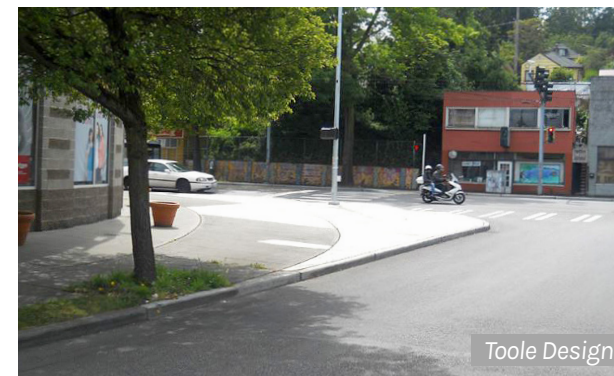
Curb radii can be adjusted to lower vehicle turning speeds
