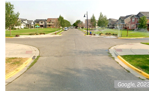
Curb extensions calm traffic in Josephine Crossing
