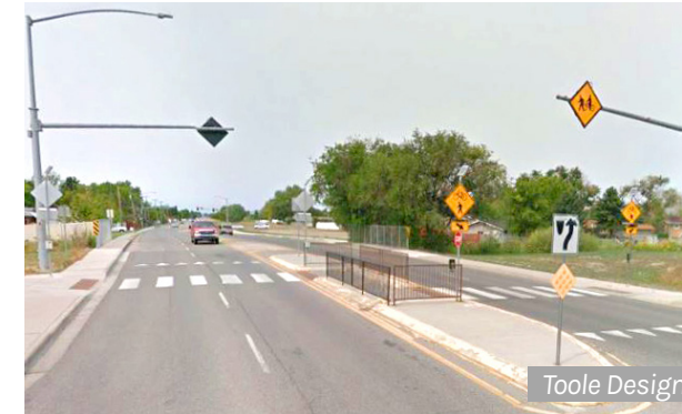
A pedestrian refuge island assists people crossing Broadwater Ave.
