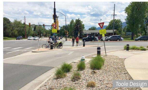
Slip lanes with added signs and raised crosswalks bring attention to pedestrians
