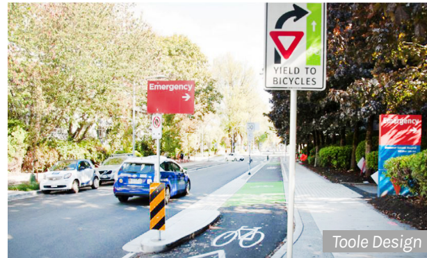
Bike-specific yield markings and signs may be necessary depending on the situation
