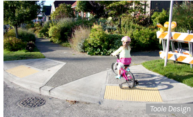
Each corner should have two curb ramps, one for each crossing
