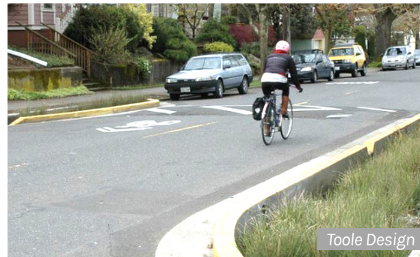
Speed humps help with traffic calming on streets that have high numbers of bicyclists
