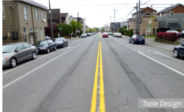
A three-lane to two-lane reconfiguration
