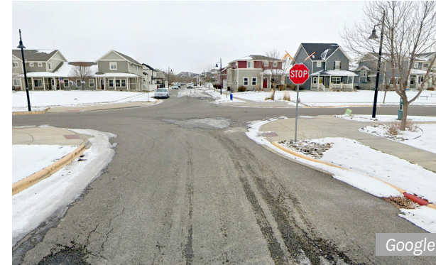
A new stop sign supplements curb extensions in Josephine Crossing
