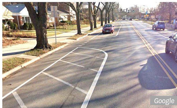
A protected bike lane created with a lane reconfiguration and re-striping
