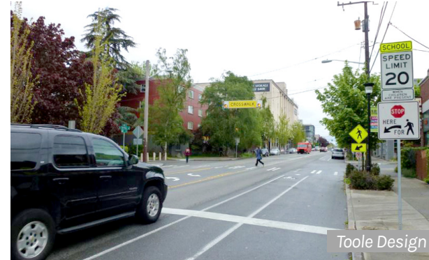
Advanced stop bars increase visibility of people crossing the street
