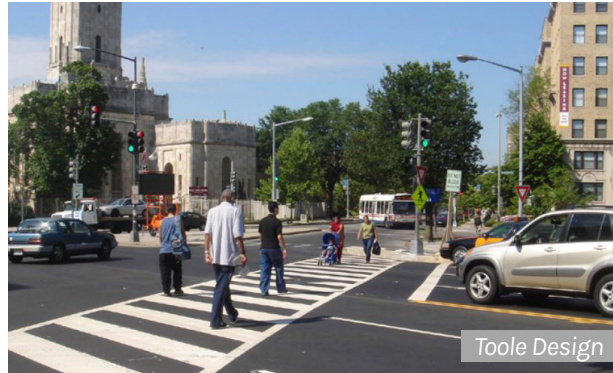
Marked ladder style crosswalk at an intersection
