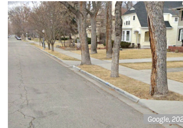
This sidewalk on Clark Ave. is separated and, because of the curb and frequent street trees, has a higher level of protection.
