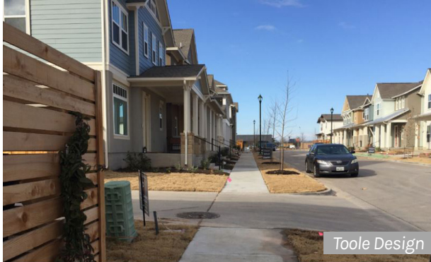
New sidewalk remains level across driveway
