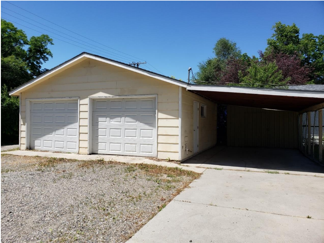
Photo 5: Detached Garage & Carport Photographer Facing: West
