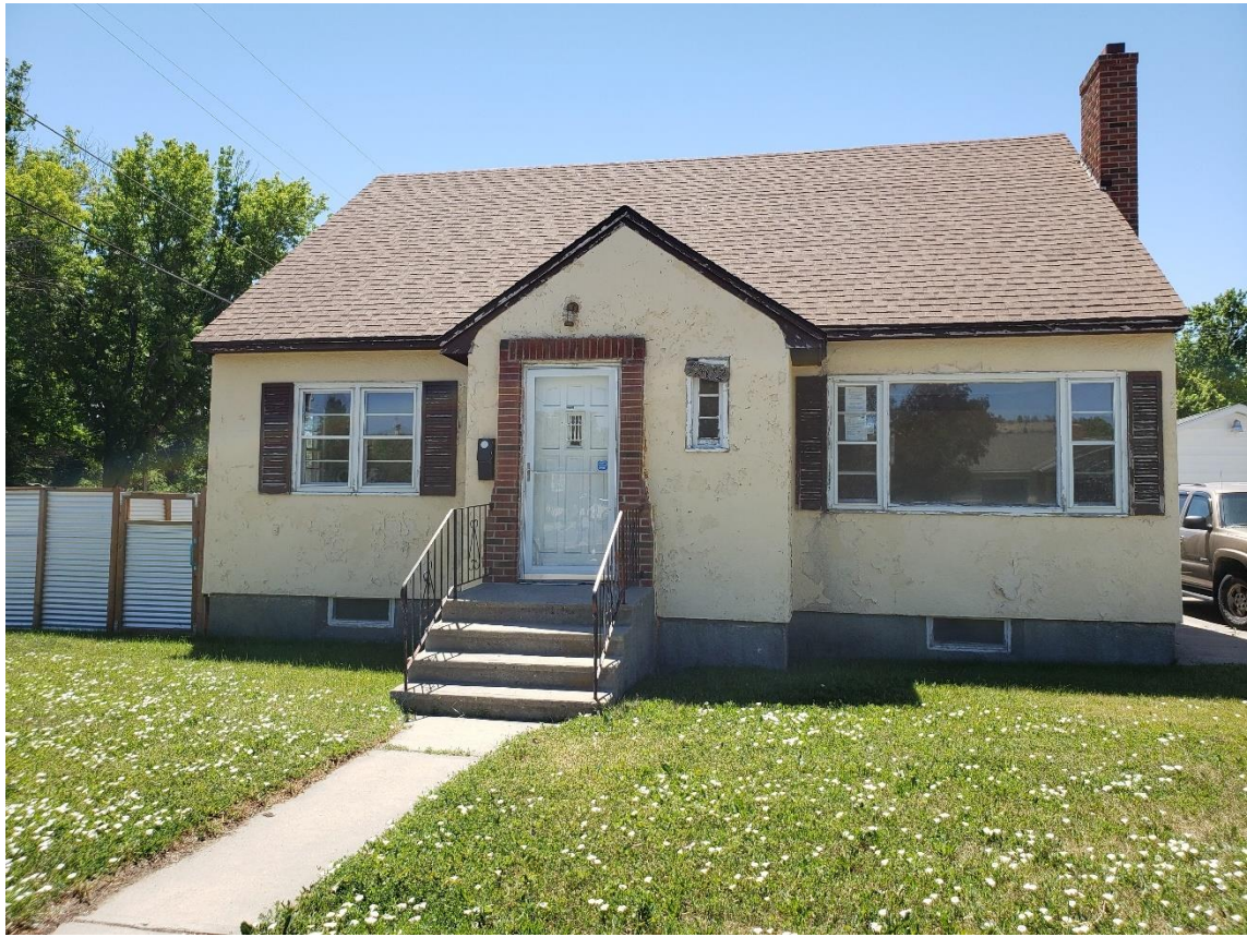
Photo 1; Front Façade Photographer Facing: South
