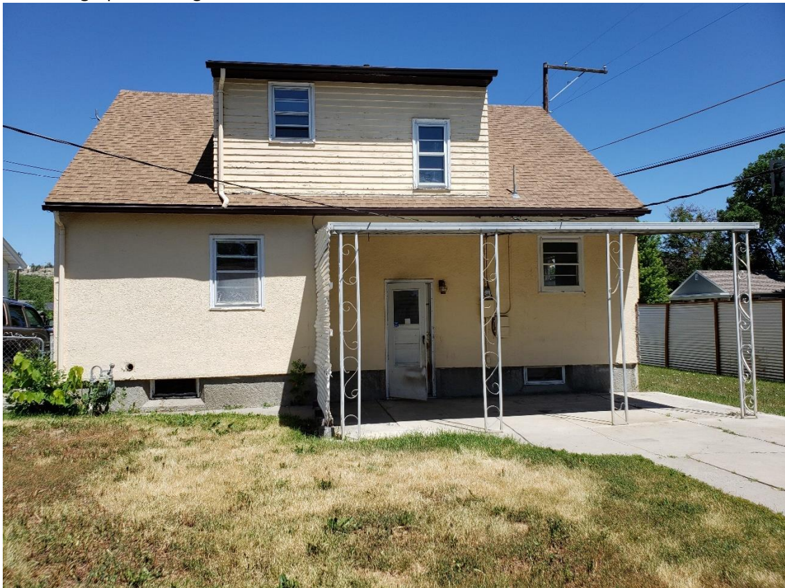
Photo 2; Rear Façade Photographer Facing: North
