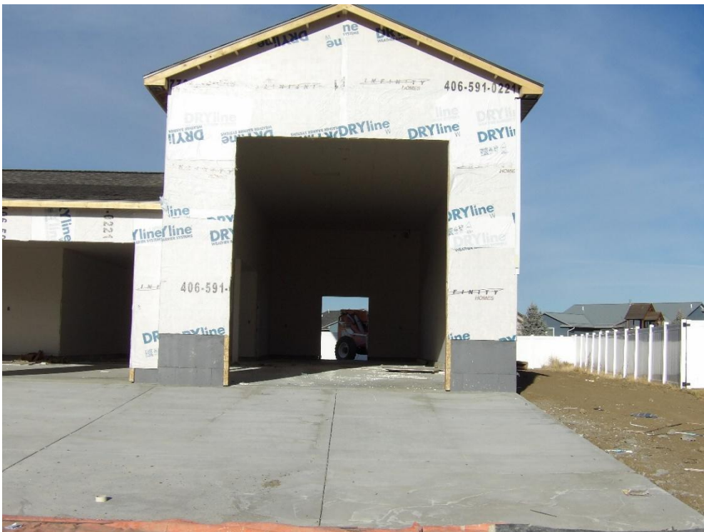
Close up of oversized shop
