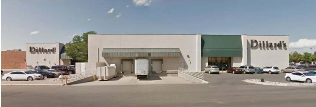
Dillard's Signage- two signs on a side elevation facing Phyllis Lane - 430sf total
