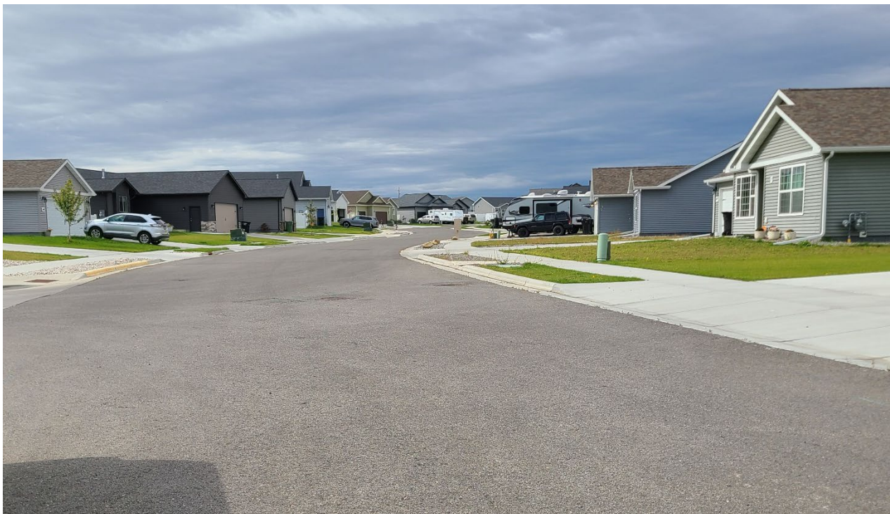
View west from current dead-end of Las Palmas
