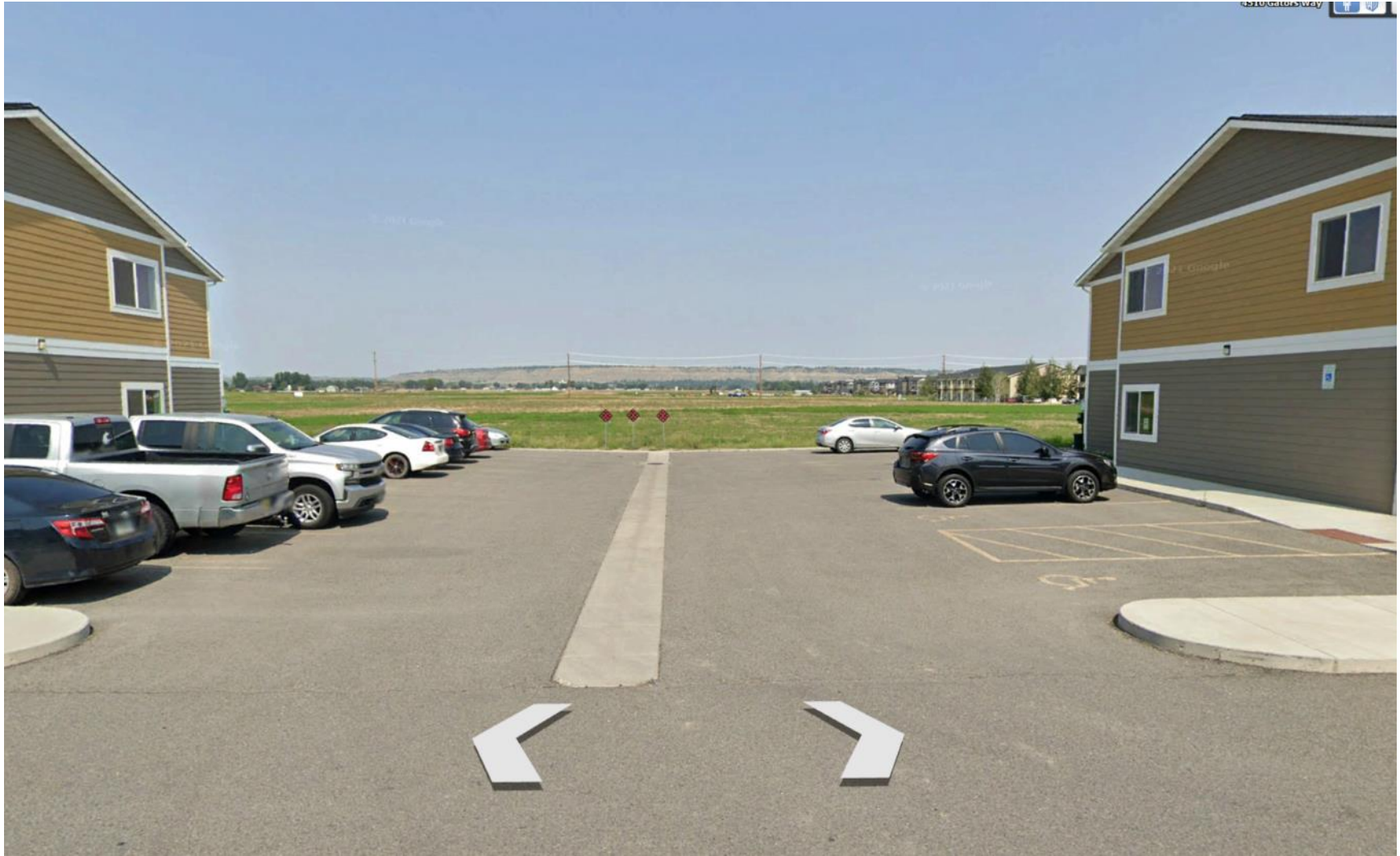
Figure 4: View looking north from property to south.
