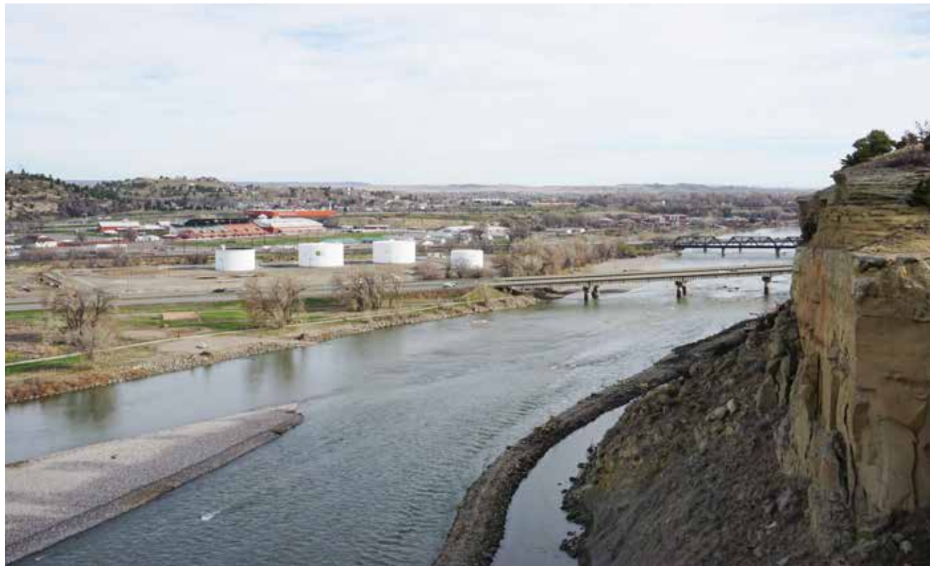
I-90 Bridge crossing over Yellowstone River - slated for replacement by MDT
