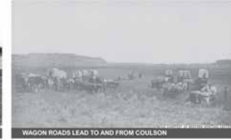
WAGON ROADS LEAD TO AND FROM COULSON
