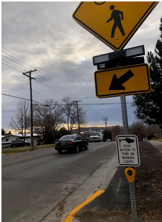
This is a similar Rapid Flashing Beacon Pedestrian Crossing installation at Virginia Lane and Avenue E to what would be installed on Montana Avenue.
