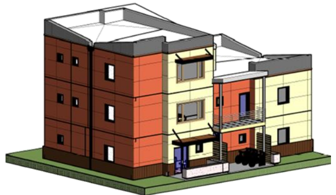
6 3D-SPLEX EXTERIOR FRONT VIEW 1
