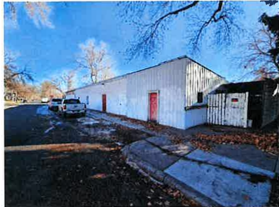
3) Meat House and Lockers building looking southeast. All substrates tested negative for lead.
