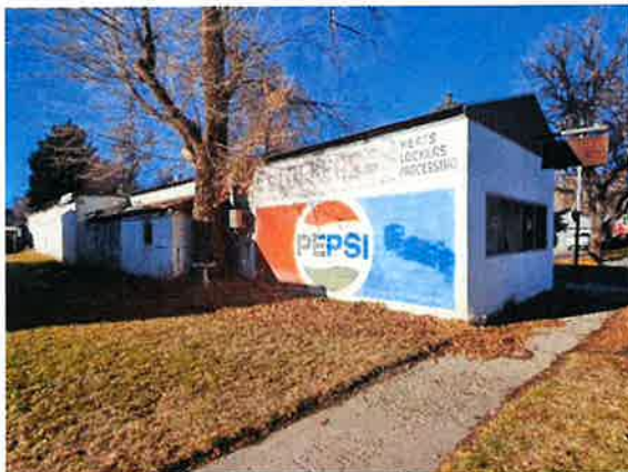
2) Meat House and Lockers building looking northwest. Red paint of the Pepsi logo tested positive for lead. One 5-point composite soil sample was collected underneath the logo. Window glazing positive for asbestos on the east facing windows.
