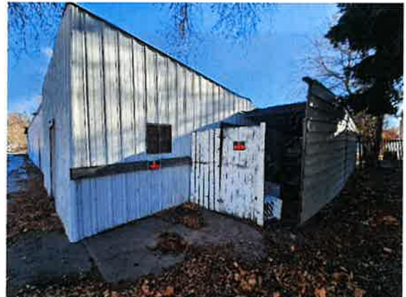
8) Photograph of the east end of the building. Exterior corrugated sheet metal siding is negative for lead.
