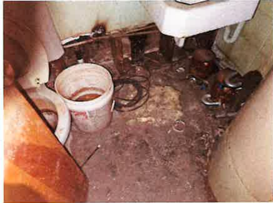
19) Photograph of the eastmost bathroom. Sheetrock materials contain <1% asbestos.
