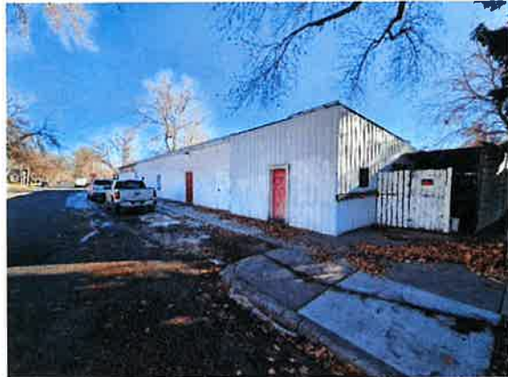
3) Meat House and Lockers building looking southeast. All substrates tested negative for lead.
