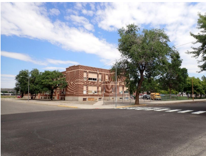
The Garfield School has been repurposed for alternative use, which may not be the most efficient use of the structure without extensive remodeling and retrofitting.
