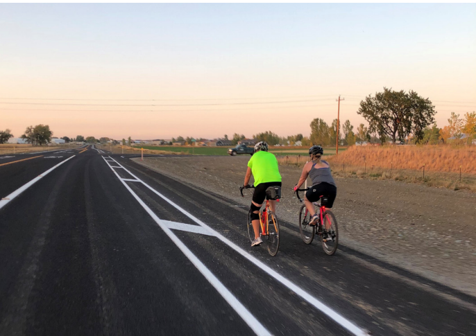
Buffered bicycle lane. Source: DOWL
