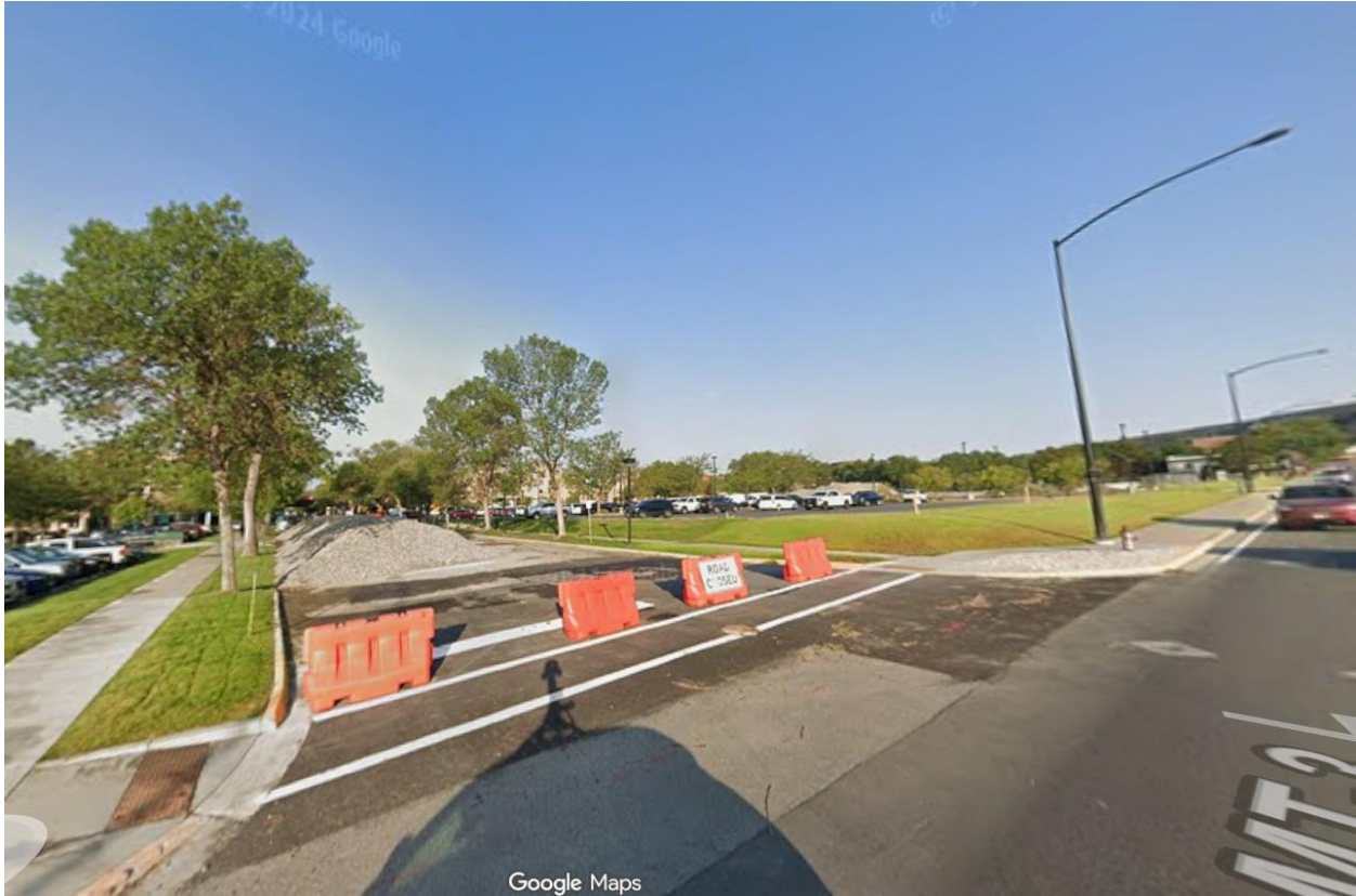
Google image just prior to beginning of construction.
