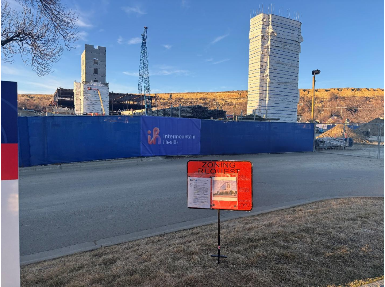
View looking north west at current construction.
