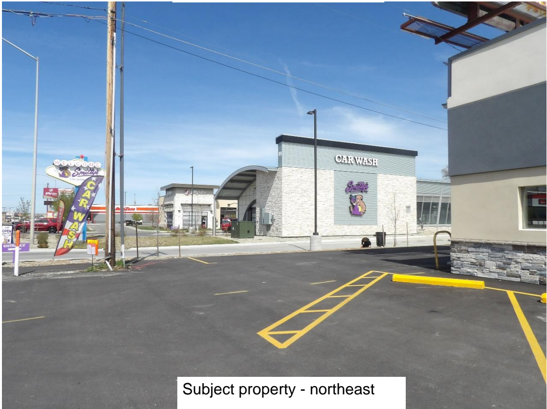
Subject property - southeast
