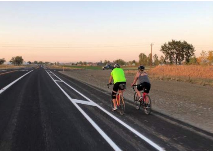
Buffered bicycle lane. Source: DOWL
