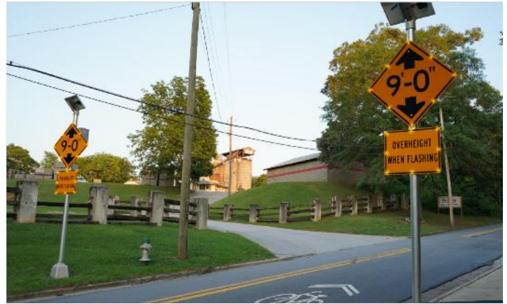
FIGURE 9. EXAMPLE OF A VERTICAL CLEARANCE WARNING SYSTEM
