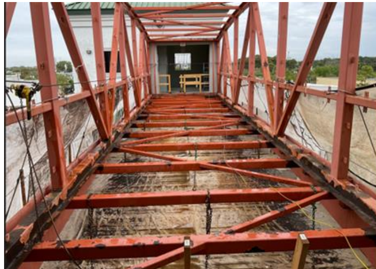
Pedestrian Bridge Rehabilitation
