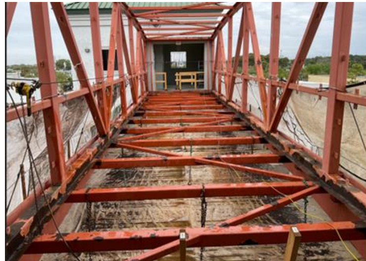
Pedestrian Bridge Rehabilitation
