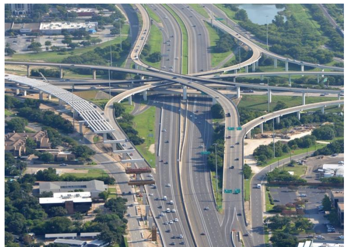
Construction at the MoPac/US 183 Interchange
