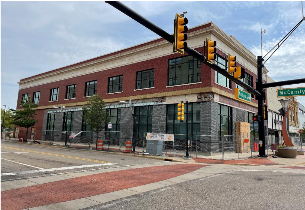
Current (under construction)
