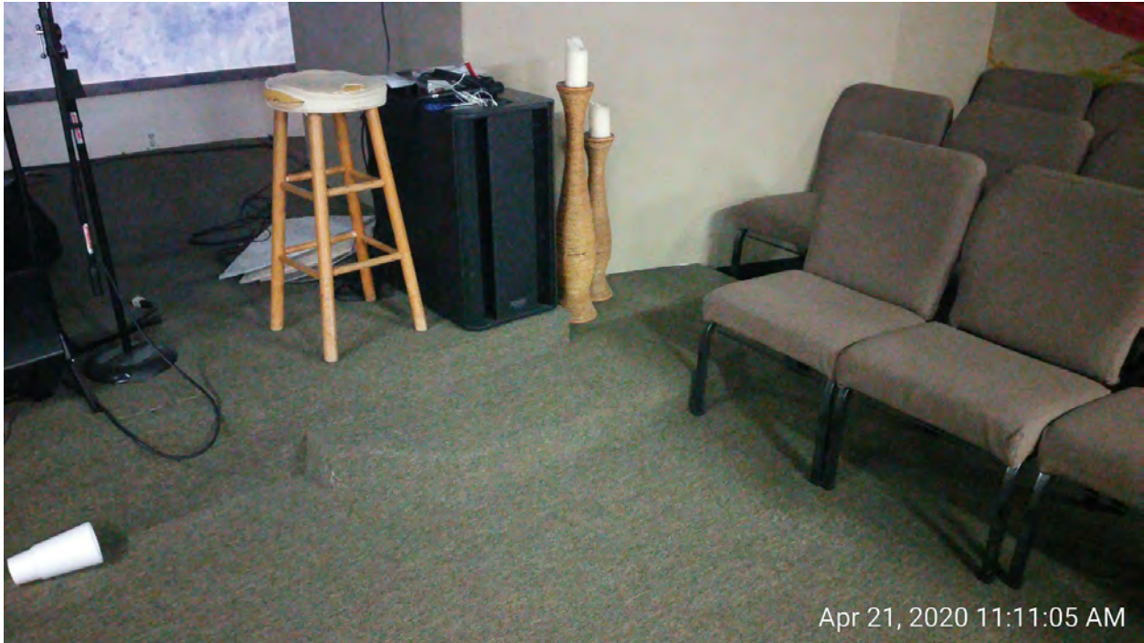
Stairs from sanctuary to stage are not accessible. Contrasting stripe required at top of stairs and bottom tread and no handrail is in place. N
