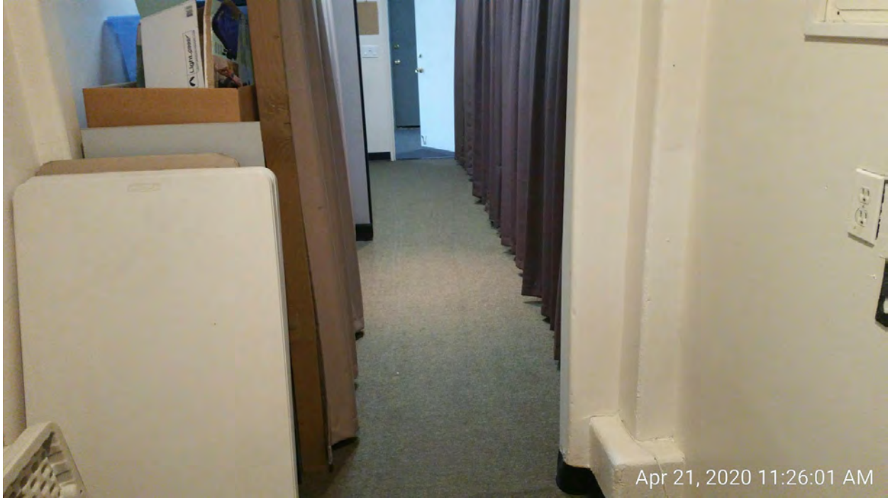
Aisle widths are too narrow at “back of house” area. E
