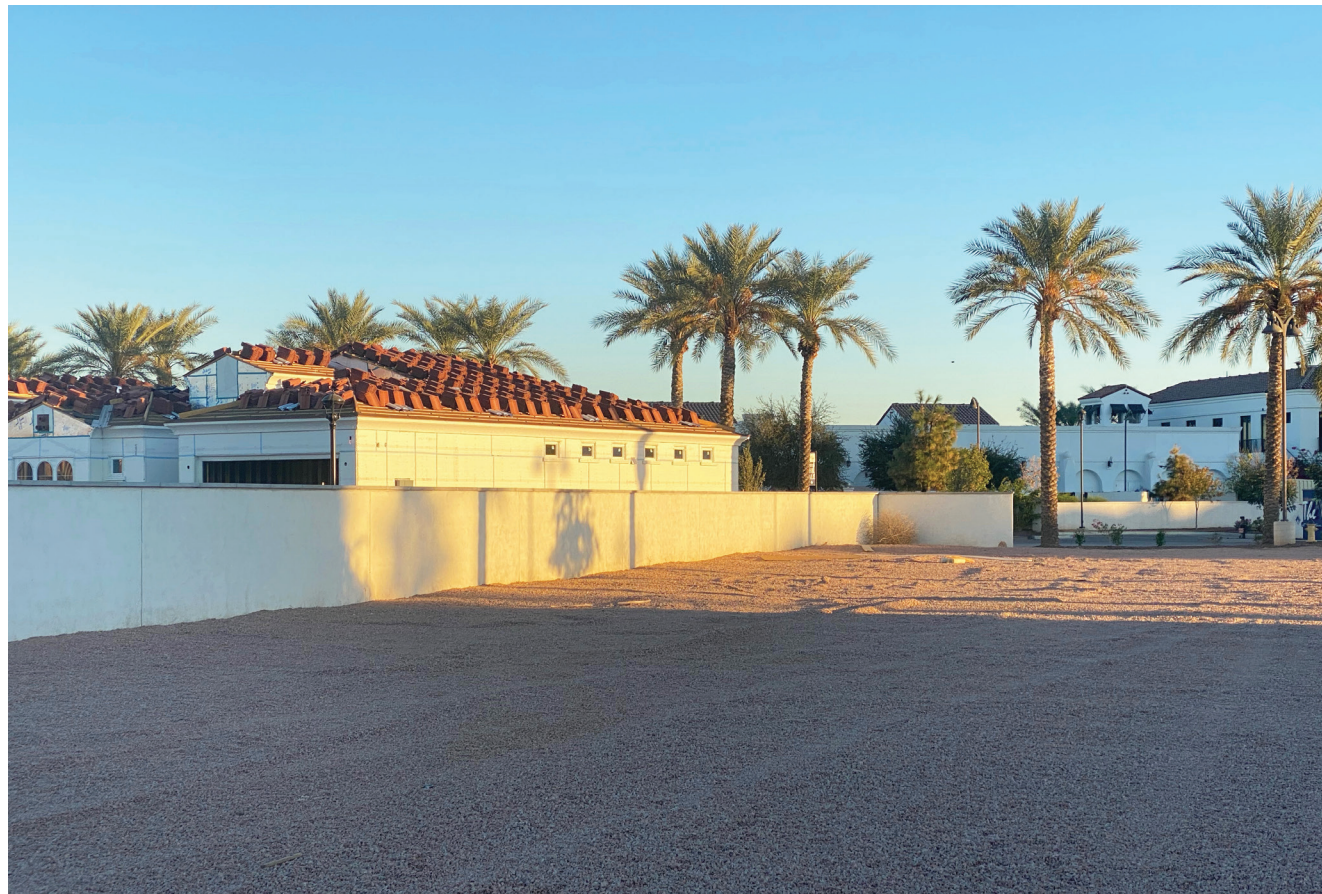
6' HIGH CMU WALL WITH STUCCO FINISH BOTH SIDES PAINTED WHITE
