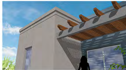
patio and window shade trellis
