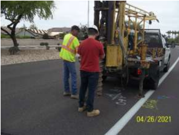
Dobson Rd @ B-3, looking south.
