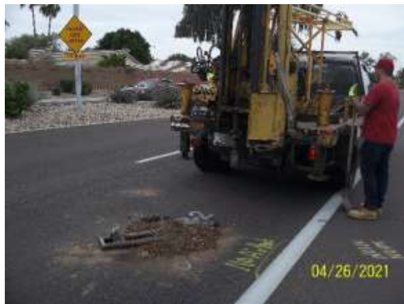
Dobson Rd @ B-2, looking south.
