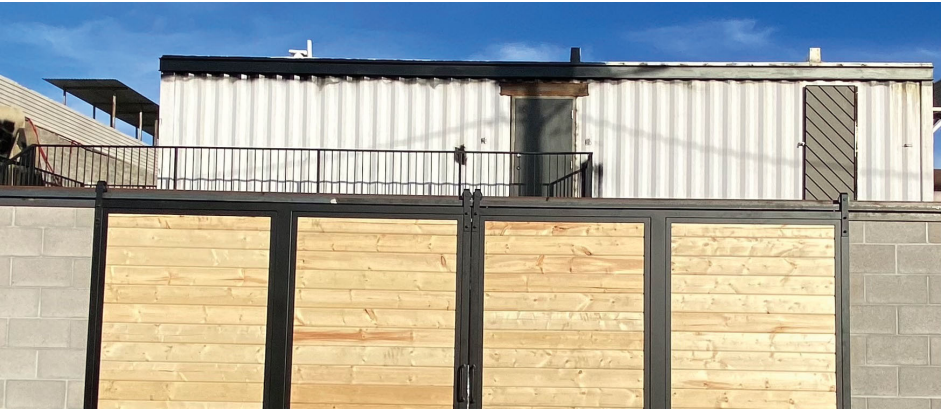
Current conditions of shipping container
