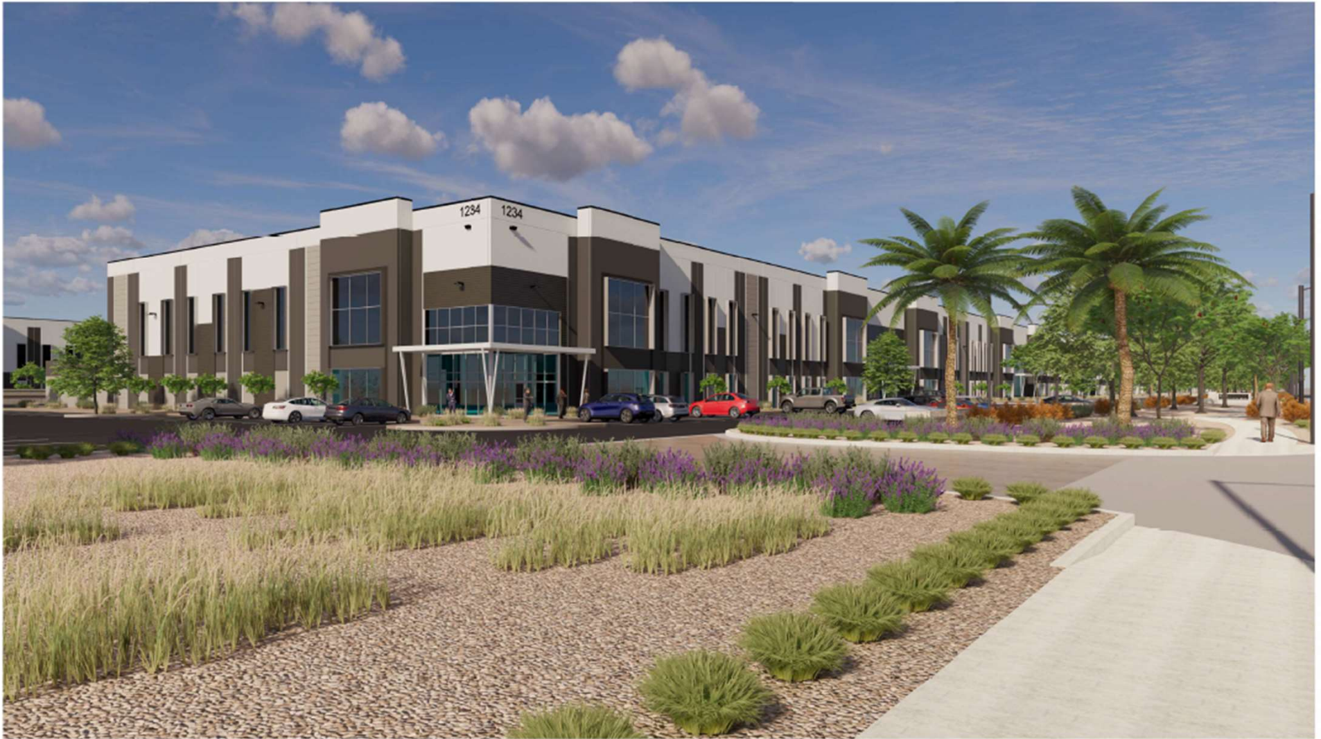
RYAN COMMERCE CENTER: NORTHEAST LOOKING SOUTHWEST
