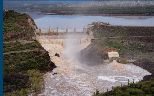
Horseshoe Dam – Verde River
