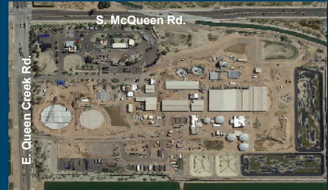
Airport Water Reclamation Facility
