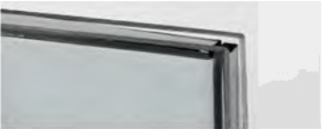
STOREFRONT GLAZING SYSTEM: VITRO ARCHITECTURAL GLASS SOLARGRAY (2) SOLARBAN 60 (3) CLEAR WITH REFLECTIVE COATING
