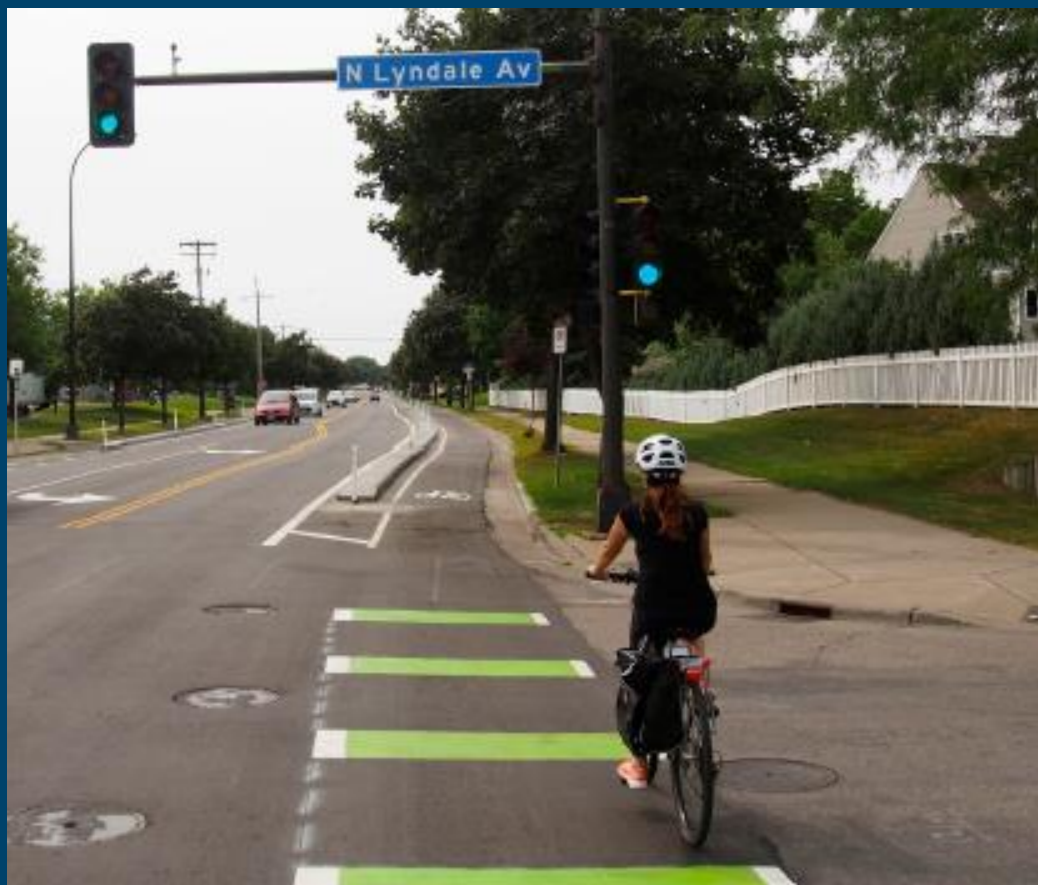
Photo Source: Minneapolis Public Works
