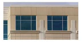
PPG PACIFICA - 1 " INSULATED GLASS SOLARBAN 60 (3) U-VALUE OF 0.29 AND SHGC OF 0.25 CLEAR ANODIZED FRAMES AND INFILL PANELS, TYPICAL
