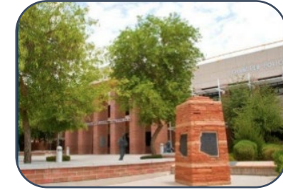
Main Station Renovations $9.6M
