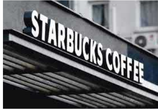
Standing Canopy Sign is a sign mounted to the top of the leading edge of a canopy located above a storefront parallel to the building façade on which it is mounted.
