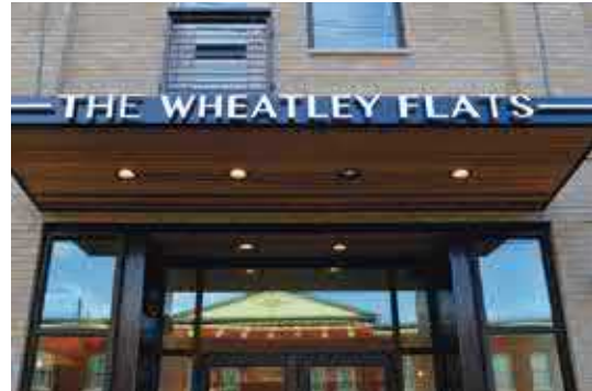
Canopy Fascia Sign is a sign attached to the vertical front face of a canopy, roof overhang, covered walkway, covered porch, or purlin of an open lattice structure.
