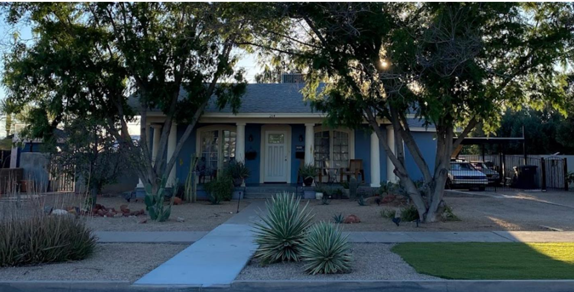
West (front) view from the street
