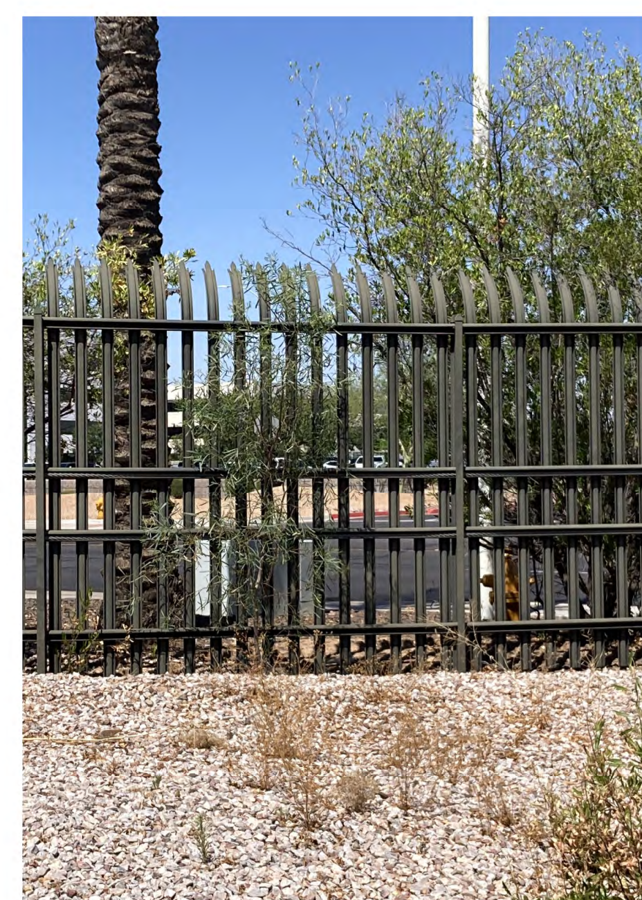
EXISTING SITE PERIMETER FENCE
