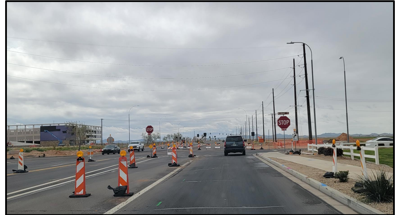
Figure 6. Gilbert Road at Hunt Highway Intersection Signal Construction Zone, March 2023
