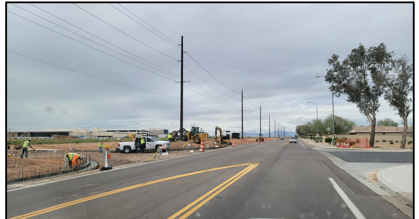
Figure 7. Existing T-Intersection being Converted to 4-legged Intersection at Santa Rita, East of Gilbert Road
