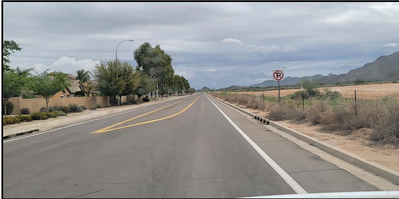
Figure 11. Existing Drainage Catch Basin Outlet
