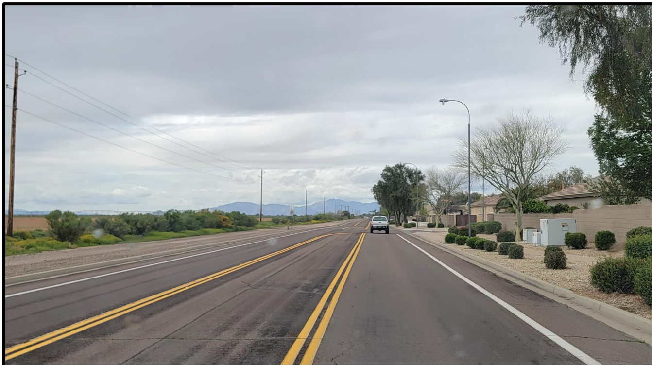
Figure 5. Existing Utility Cabinets along North side of Hunt Highway
