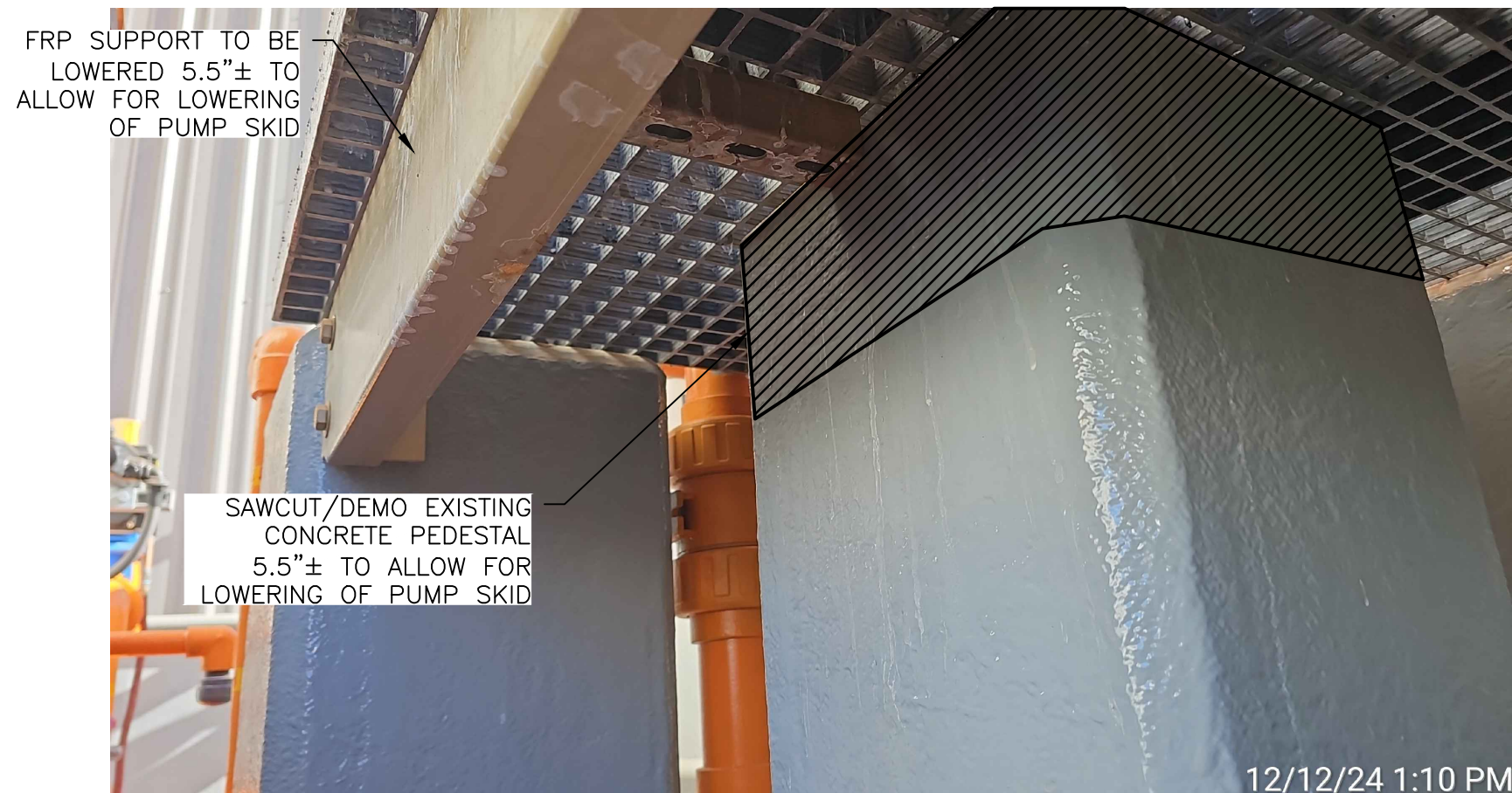
A1 EXISTING CONCRETE PEDESTAL NOT TO SCALE
