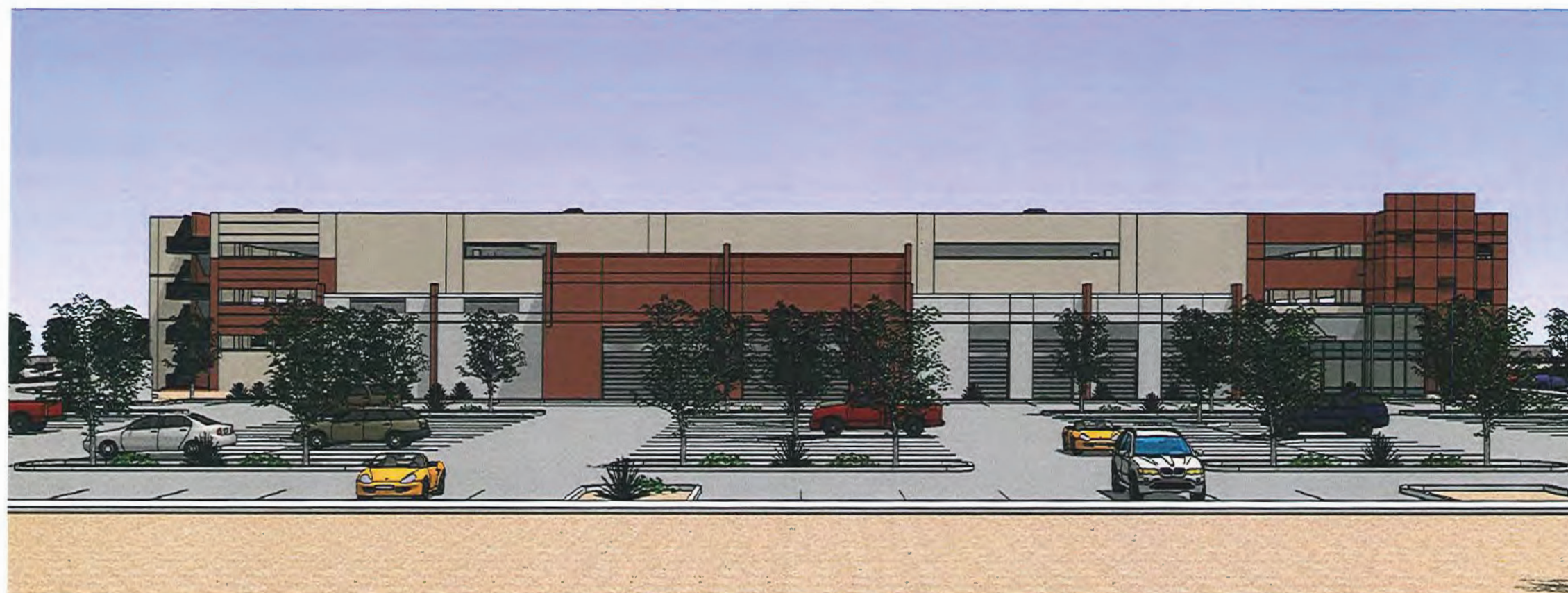
PARKING STRUCTURE LOOKING NORTH
