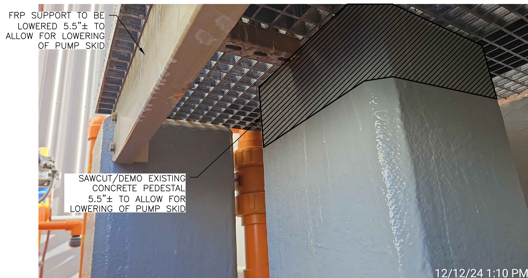
A1 EXISTING CONCRETE PEDESTAL NOT TO SCALE
