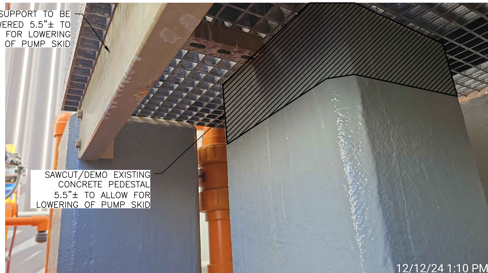
A1 EXISTING CONCRETE PEDESTAL NOT TO SCALE
