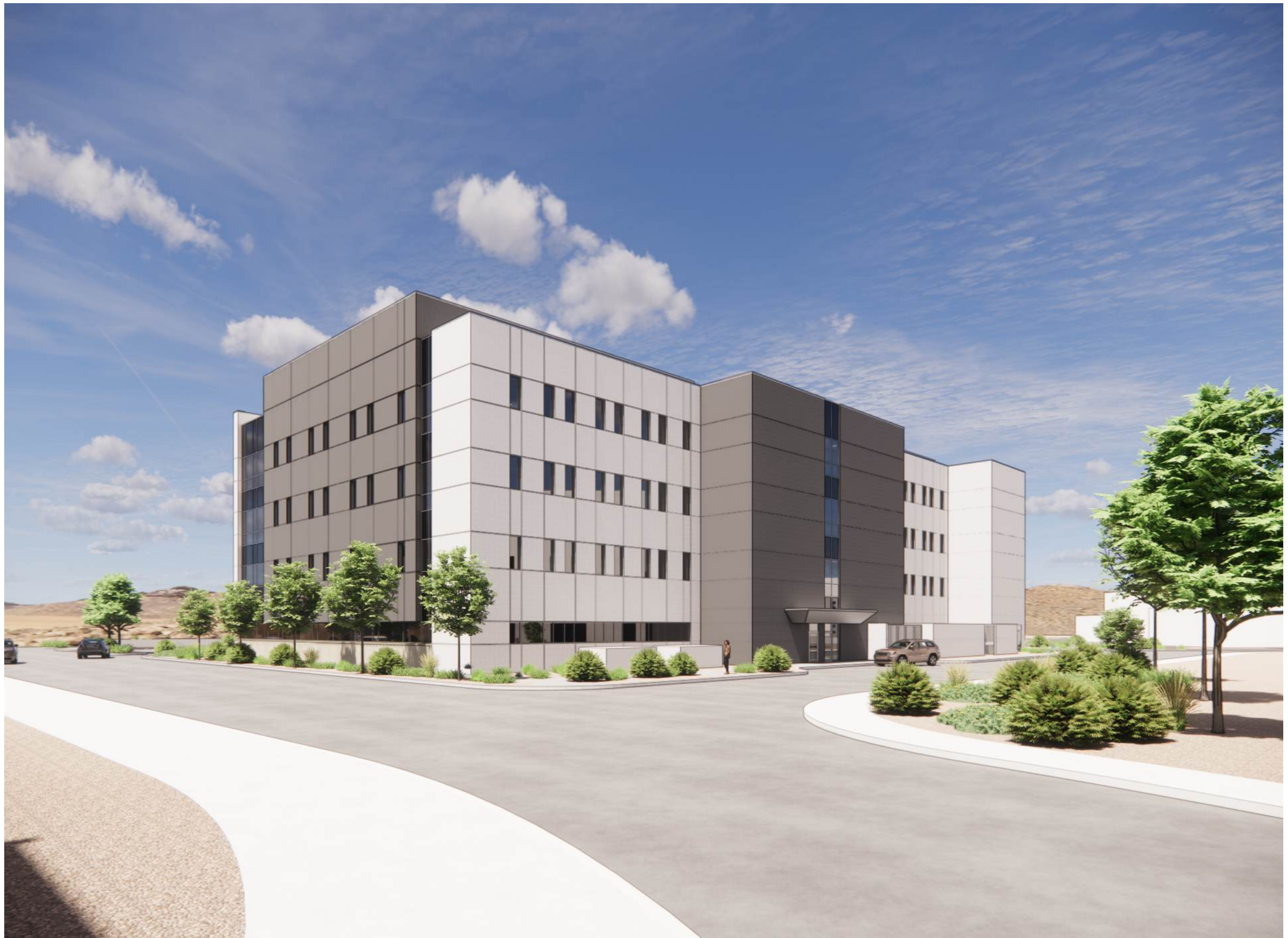
CRMC MOB - PDP - NORTHEAST CORNER
