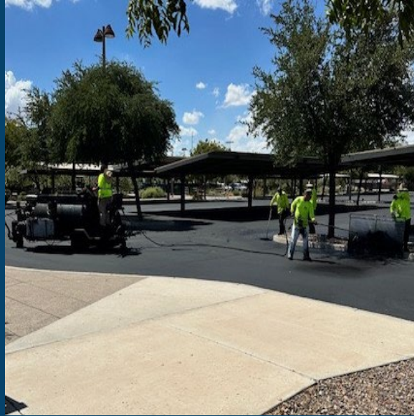
Seal Coat Applications
