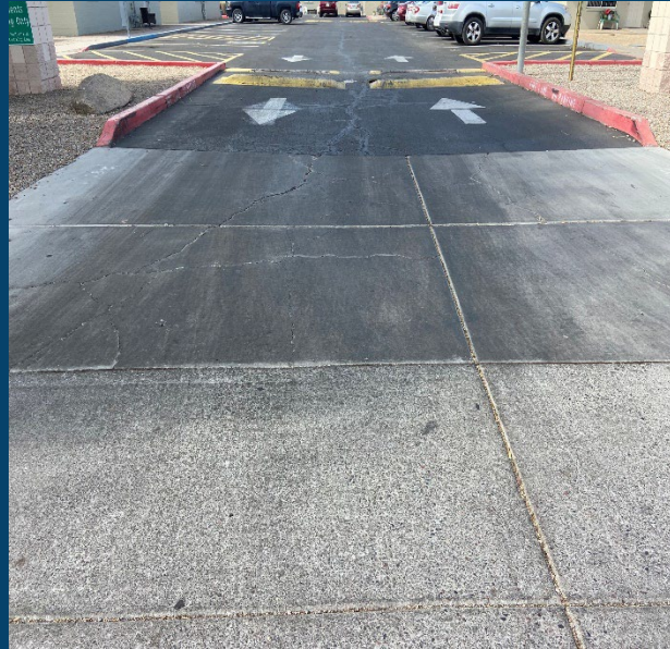
Minor Repairs and Small Area Replacement
