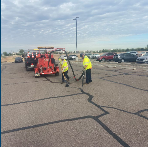
Crack Seal/Mastic Seal
