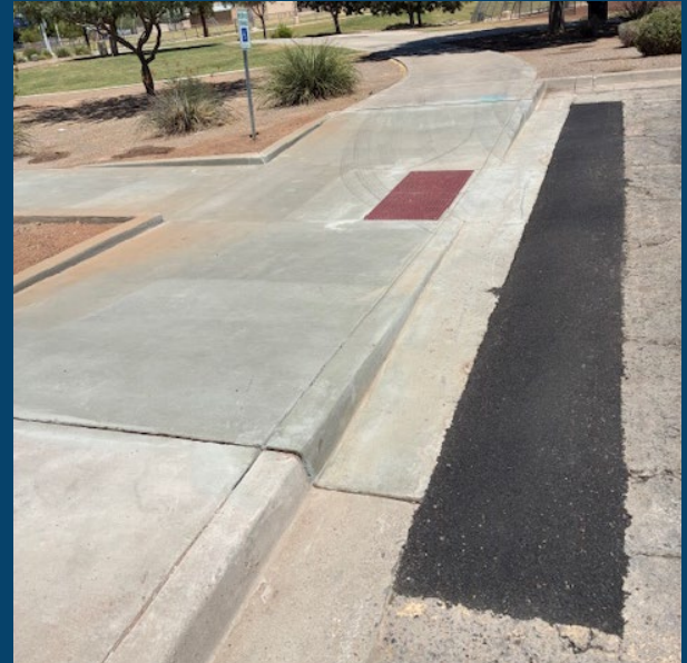
Shawnee Park ADA Ramp Replacement
