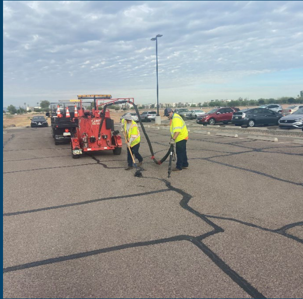
Crack Seal/Mastic Seal
