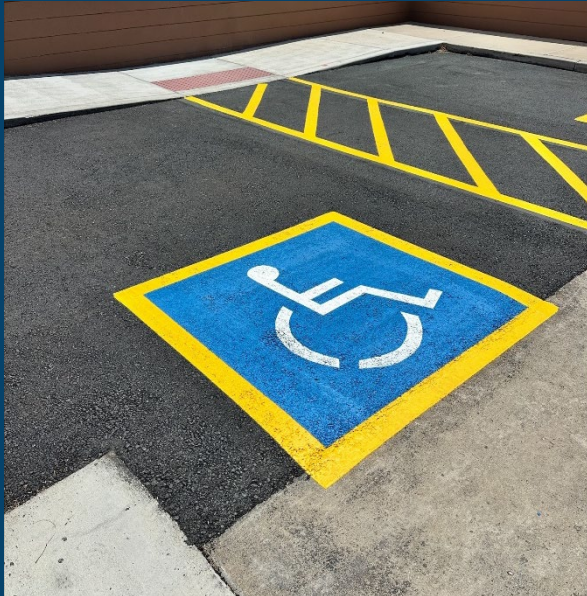
Airport Terminal ADA Ramp Replacement and Restriping
