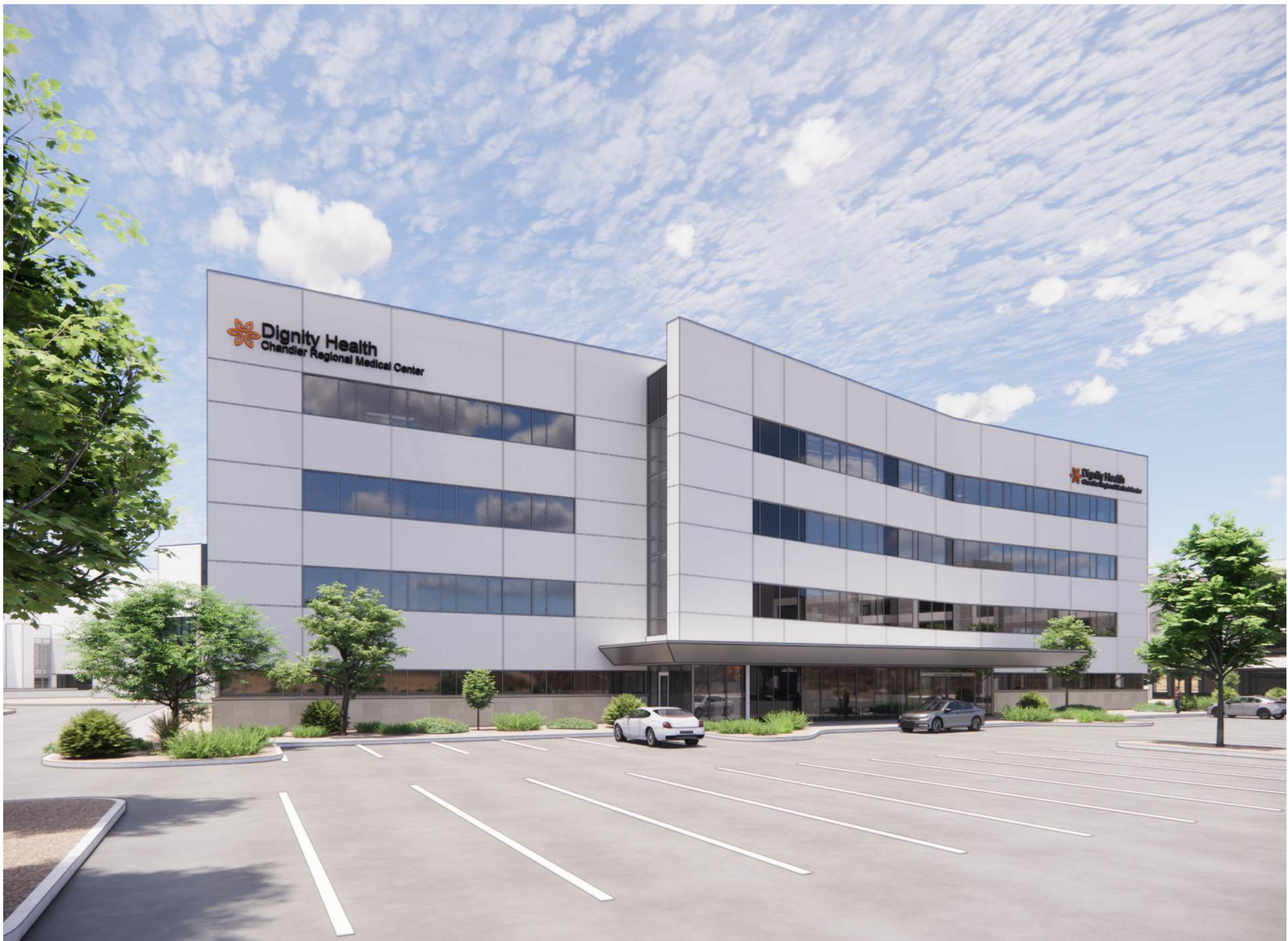
CRMC MOB - PDP - SOUTHWEST CORNER
