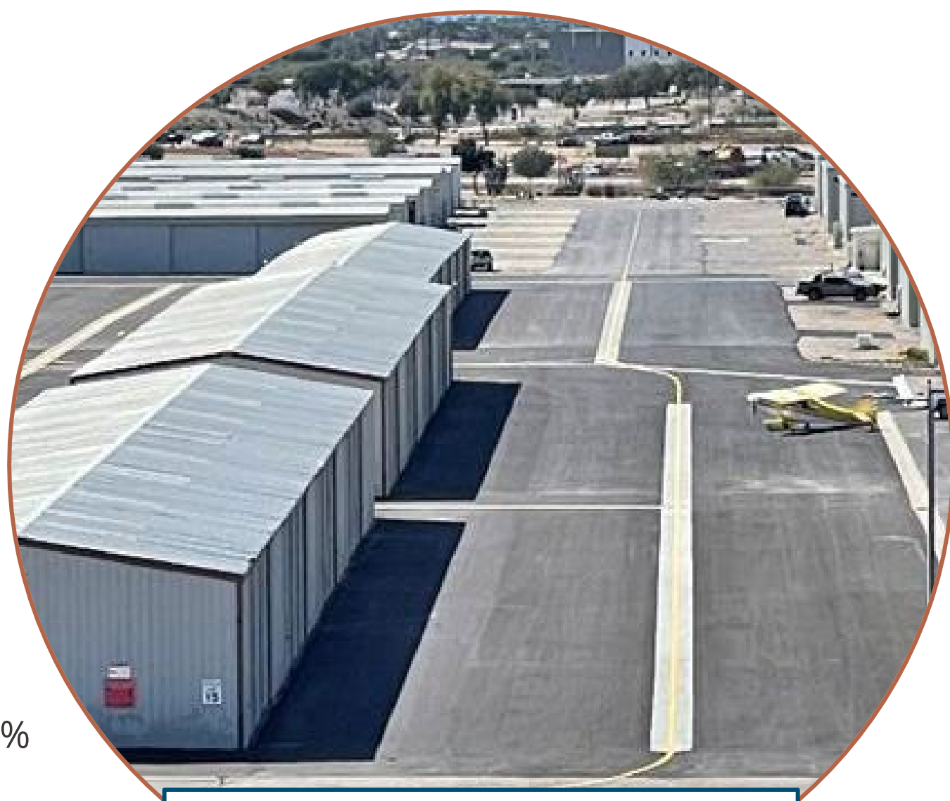
Hangar Area Pavement Replacement
