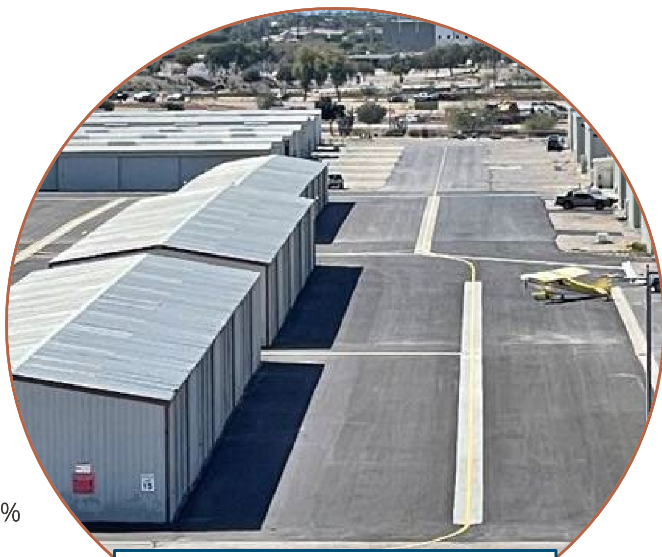
Hangar Area Pavement Replacement
