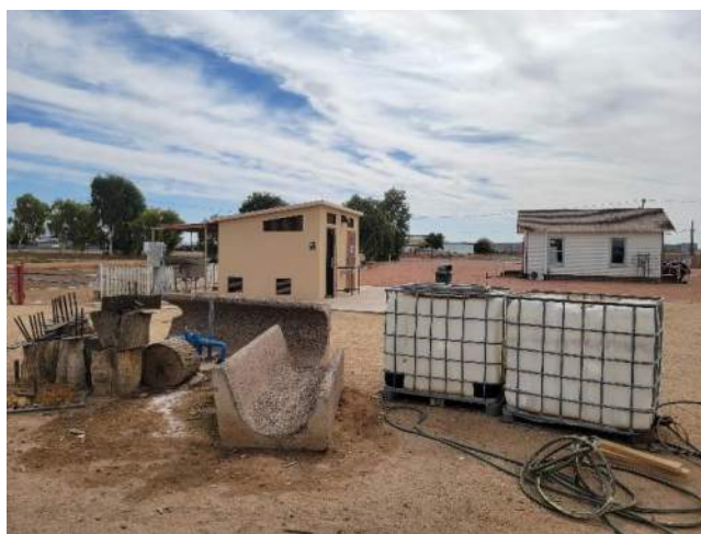
Figure 2.1.4 – View of Bathroom/Structures
