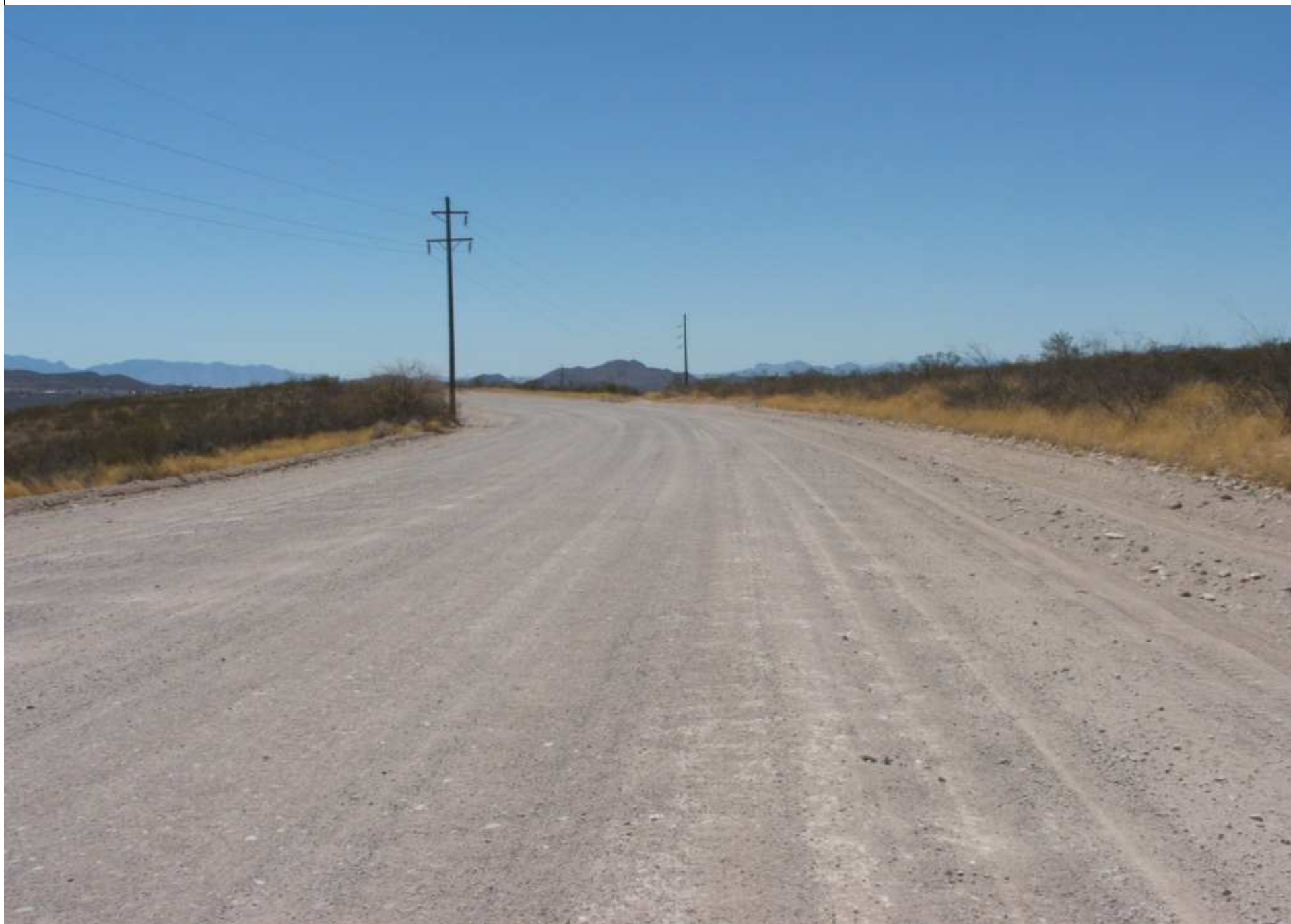
Gleeson Road (east termini) looking West.
